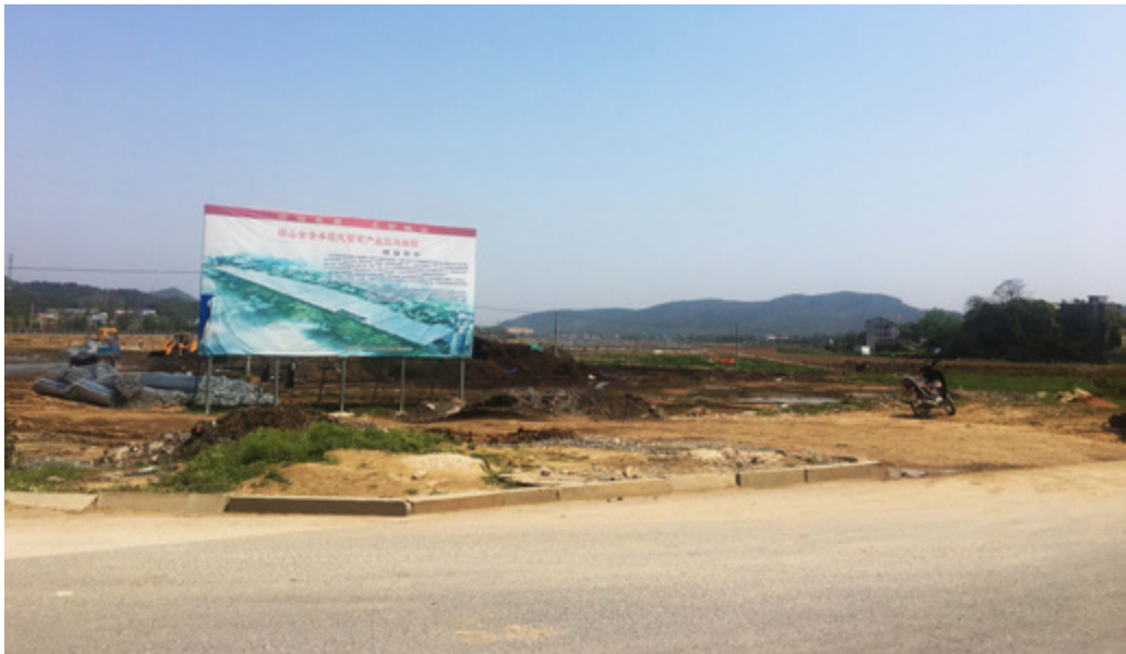
Construction of a corporate-owned modern grape farm on collective land in rural Hunan. PC: Ettore Santi.
